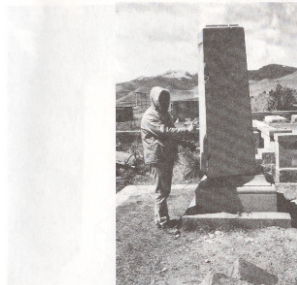
FIG. 9(a). Grave Marker That Rotated (in Spitak)
