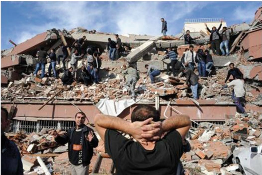
Fig. 21.1 Building collapsed during the 2011 Van Earthquake in Turkey (Courtesy of National Turk)
