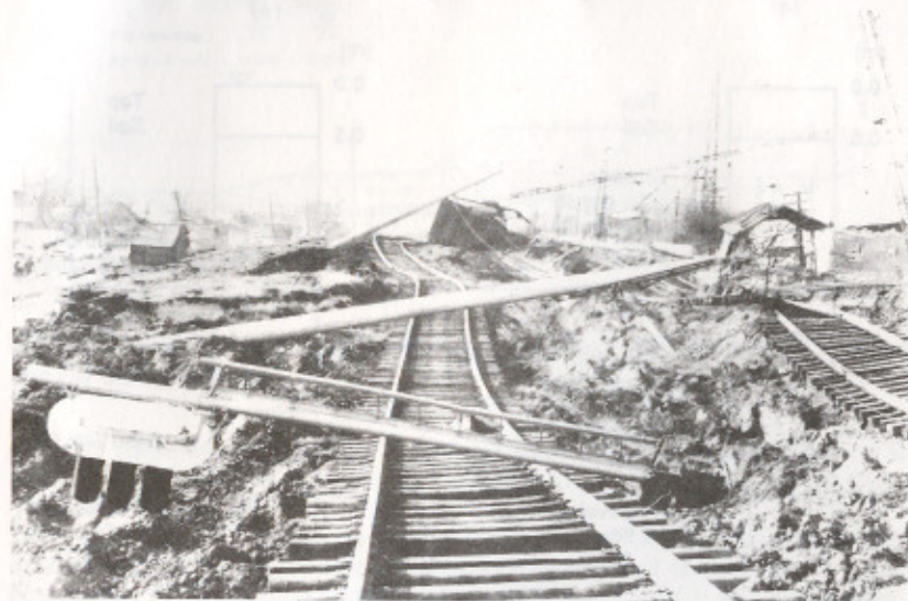
FIG. 13. Photograph of Failed Embankment at Railway Station in Nalband (Site 3) (Photo Courtesy of A. Karakhanian, 1989)
