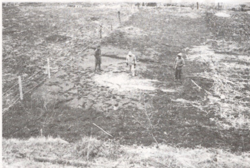
FIG. 6. Evidence of Sand Boils Adjacent to Failed Spitak Highway Embankment (Site 1)
