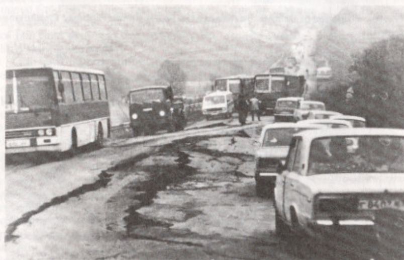
FIG. 4. Photograph of Failed Spitak Highway (Site 1)
