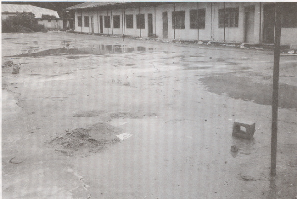
Figure 14. Photograph of a school yard in Roudboneh covered with ejected liquefied sand and water.
