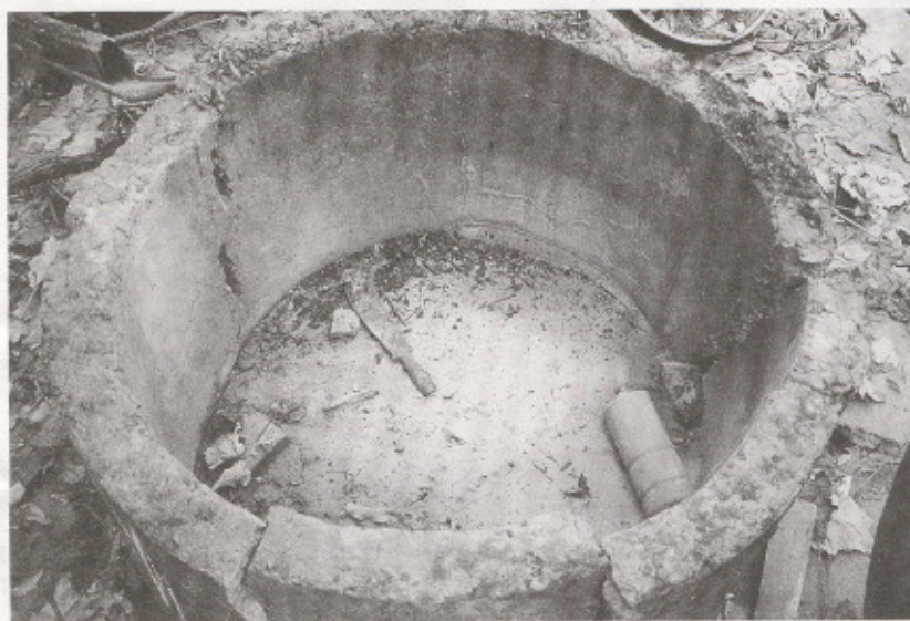
Figure 9. A water well in Astaneh-Ashrafieh filled with rising liquefied sand.
