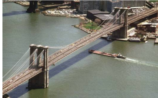
Fig. 1 Photograph of the Brooklyn Bridge.
